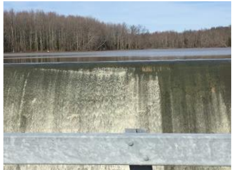
Stonelick Lake Dam
